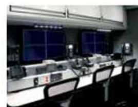
Surface Mount/Accessible Communications Wiring Raceways
